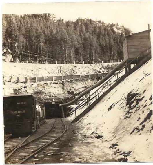
Grand Lake Tunnel
